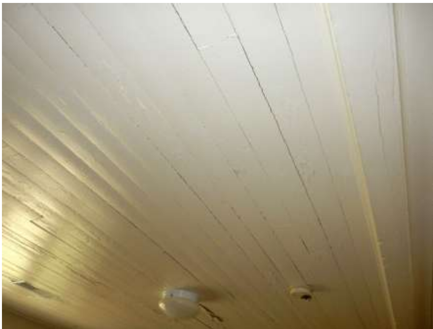
Image 59: Main Dwelling, Apartment Bead Board Ceiling, May 1, 2018
