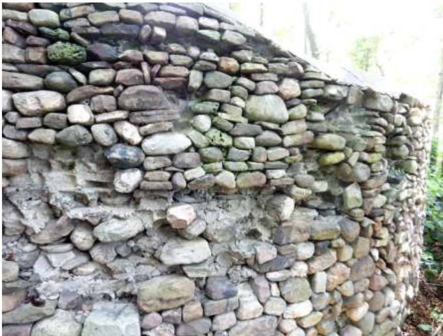
Figure 13: Cobblestone & Concrete Wall with Concrete Base Exposed, August 2017, LDW
