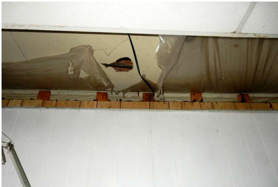
Image 28: Carriage House Apartment Bedroom, Ceiling Damage, March 6, 2018
