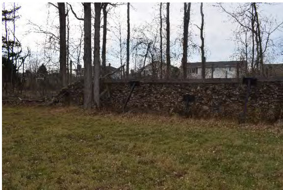
Plate 28: Partially collapsed stone wall, looking south
