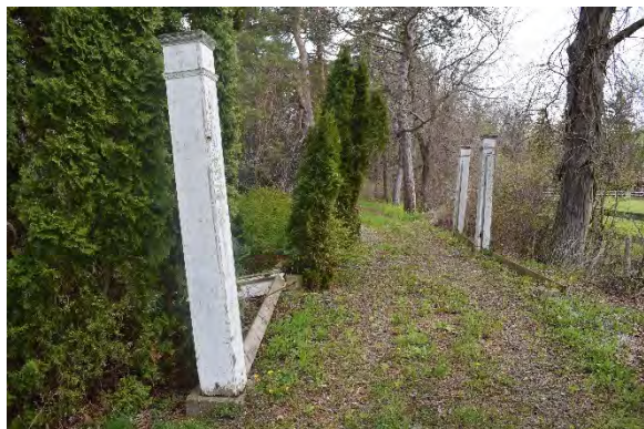
Plate 13: Looking north on access road, showing wood columns and concrete footings
