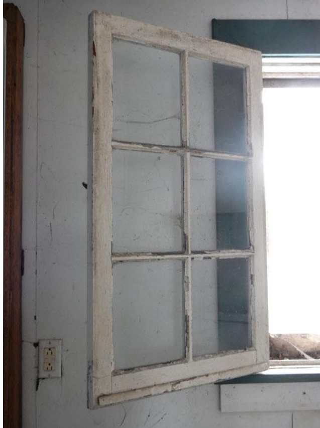
Figure 56: 200 John Street, Pool House, Casement Window
