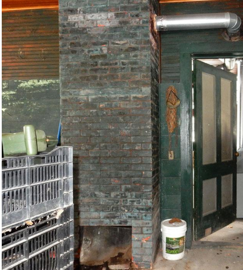
Figure24: 200 John Street, Garage, Brick Fireplace
