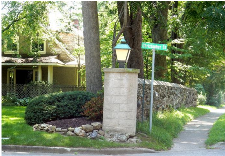
Figure29: Wall at Christopher Street and Rebuilt Pillar
