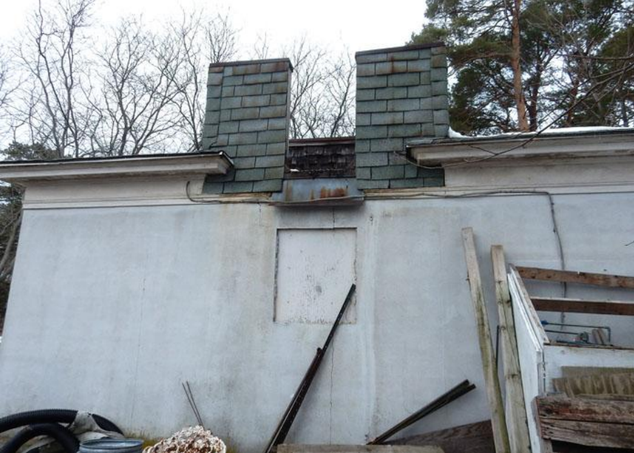
Figure 53: 200 John Street, Pool House, West Elevation
