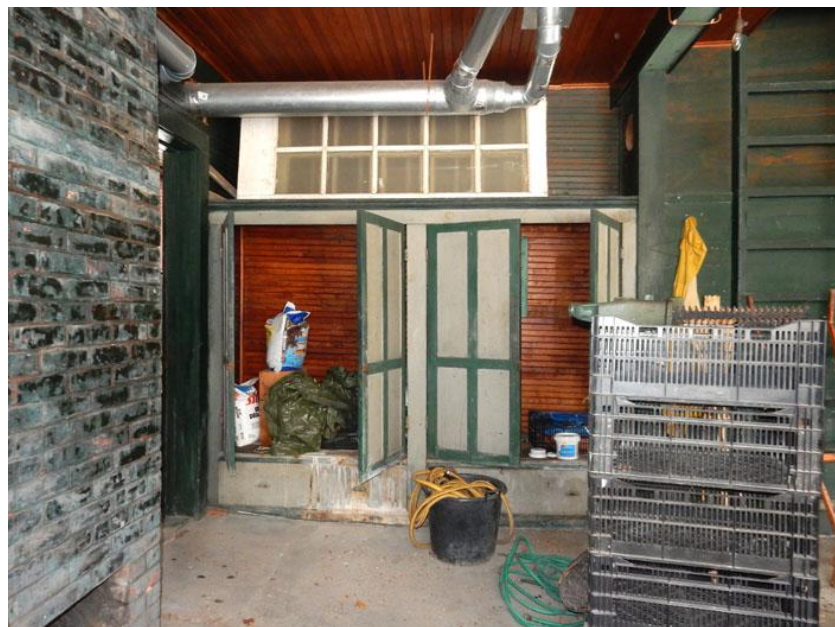
Figure25: 200 John Street, Garage, Ground Floor Storage Cupboards
