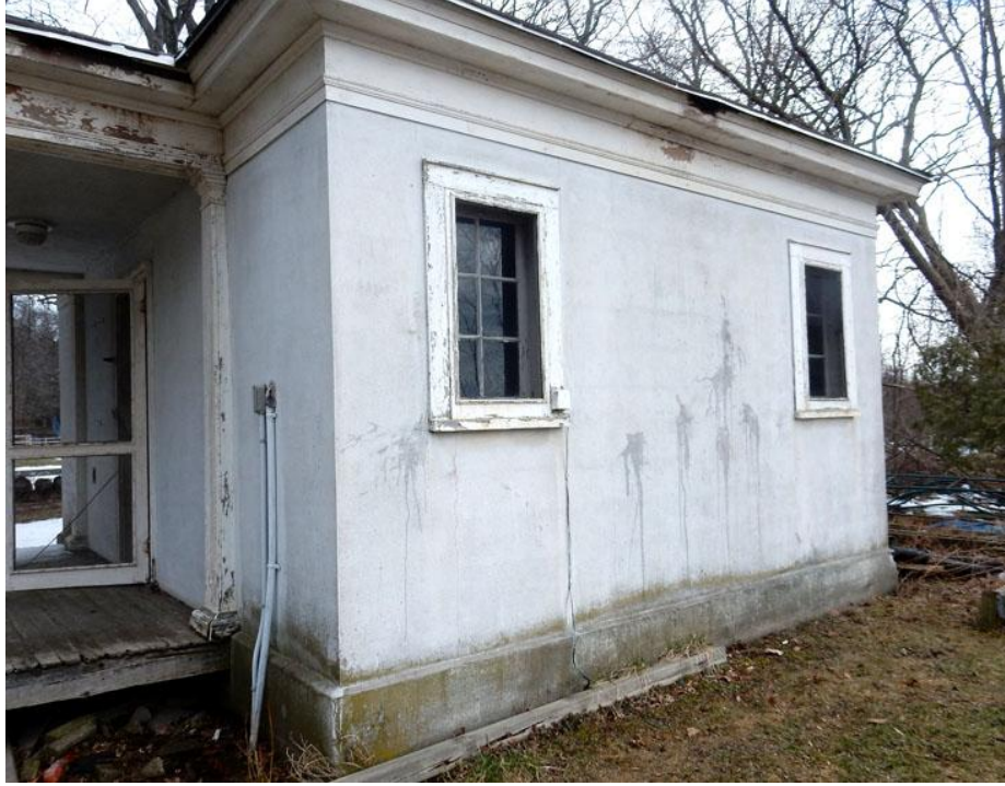
Figure52: 200 John Street, Pool House, South Elevation
