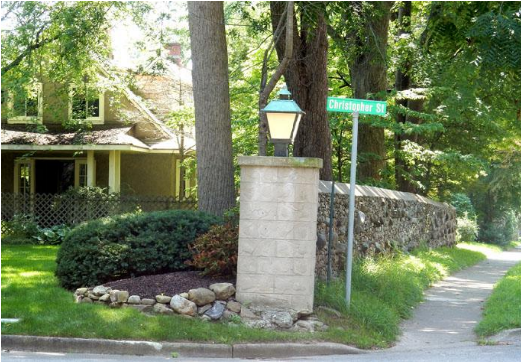
Figure 15: Rebuilt Entrance Pillar, Christopher Street
