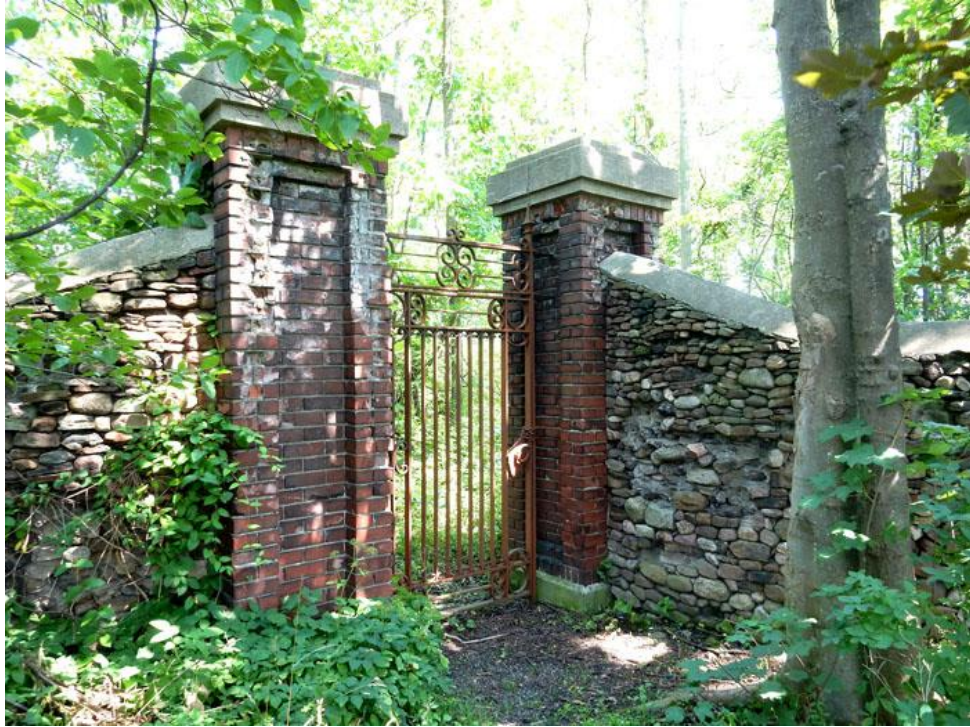
Figure60: 200 John Street, Gate & Pillars, Railway Trail
