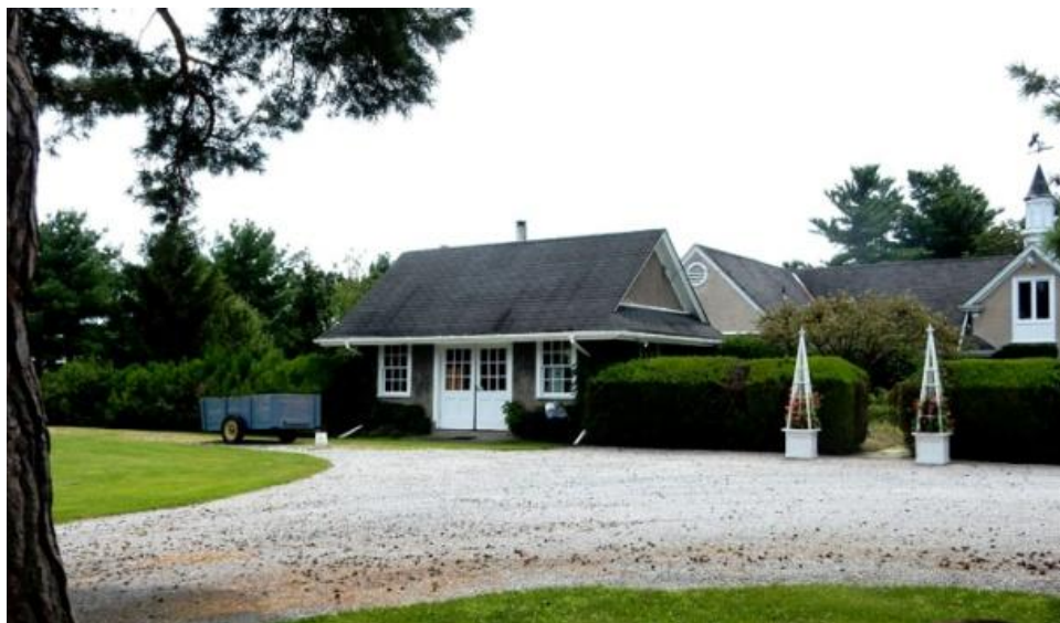
Figure25: Outbuilding at 588 Charlotte Street
