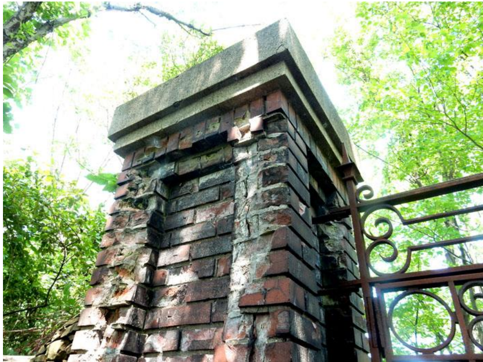
Figure61: 200 John Street, Pillar, Railway Trail
