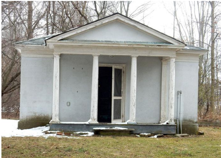
Figure46: 200 John Street, Pool House, Facade
