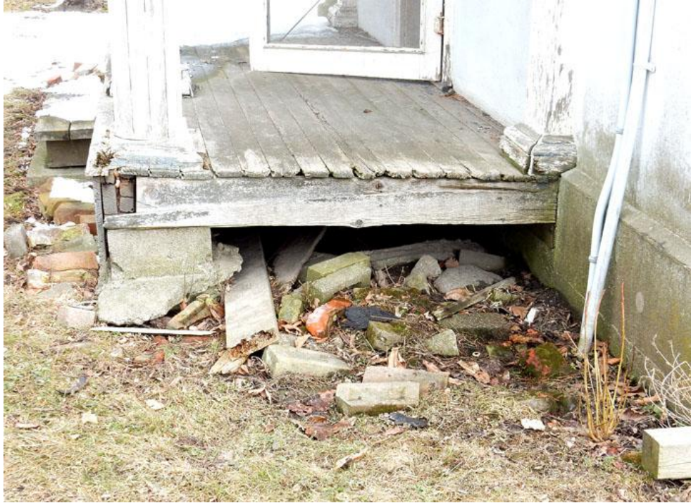
Figure50: 200 John Street, Pool House, Portico Floor
