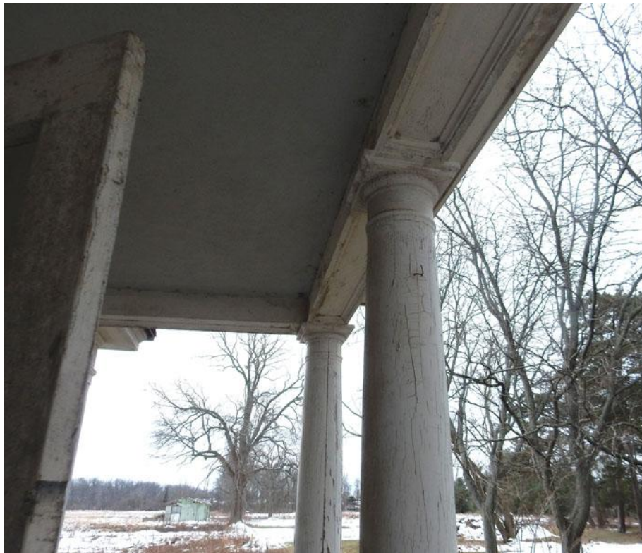
Figure49: 200 John Street, Pool House, Portico
