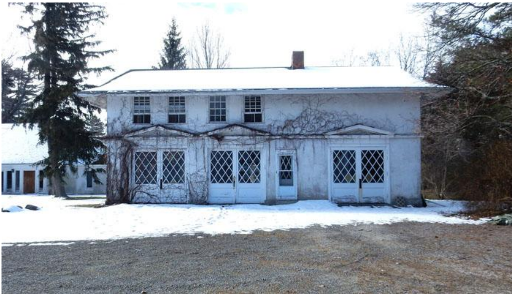
Figure 2: 200 John Street, Garage
