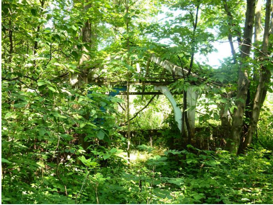
Figure 5: 200 John Street, Gazebo
