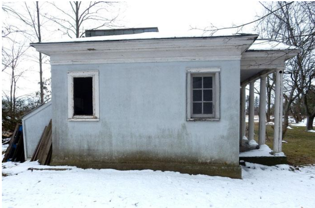
Figure51: 200 John Street, Pool House, North Elevation
