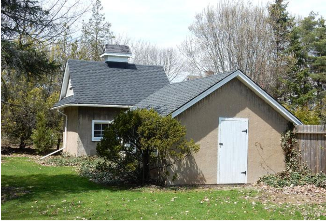
Figure86: 588 Charlotte Street, Outbuilding Three with Outbuilding One in Background
