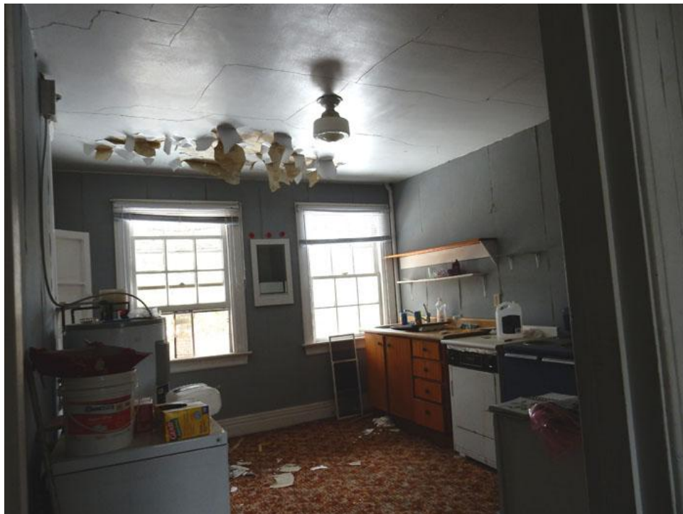
Figure27: 200 John Street, Garage, Apartment Kitchen
