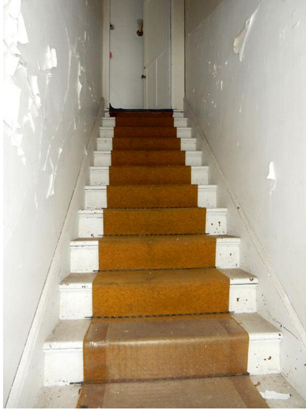
Figure26: 200 John Street, Garage, Apartment Entrance Stairs
