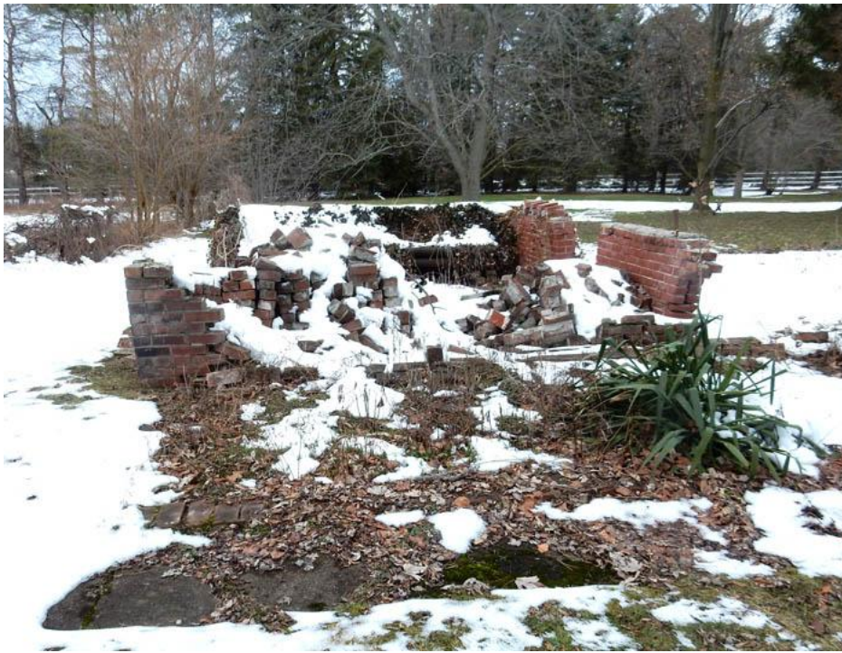
Figure 6: 200 John Street, Remnants of Greenhouse Foundation
