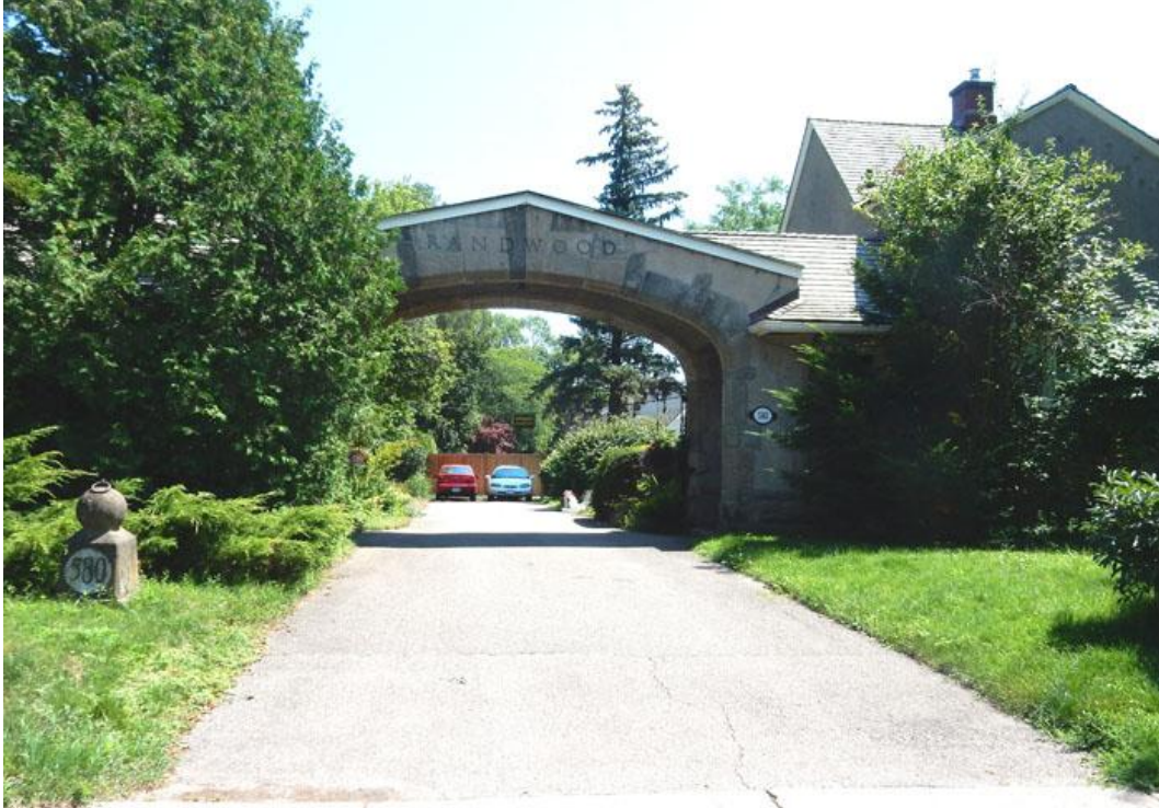
Figure 16: Stone Entrance Arch, 580 Charlotte Street
