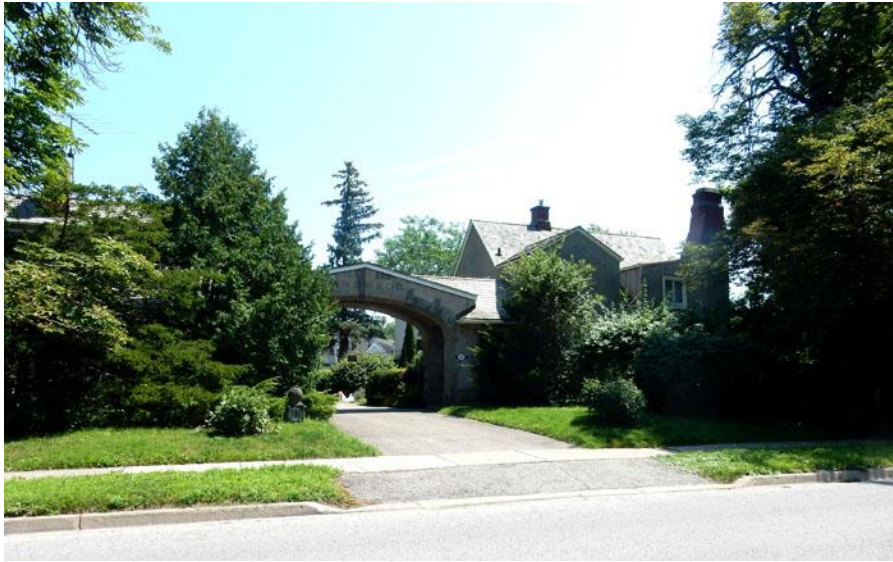
Figure28: Gatehouse and Archway, Charlotte Street
