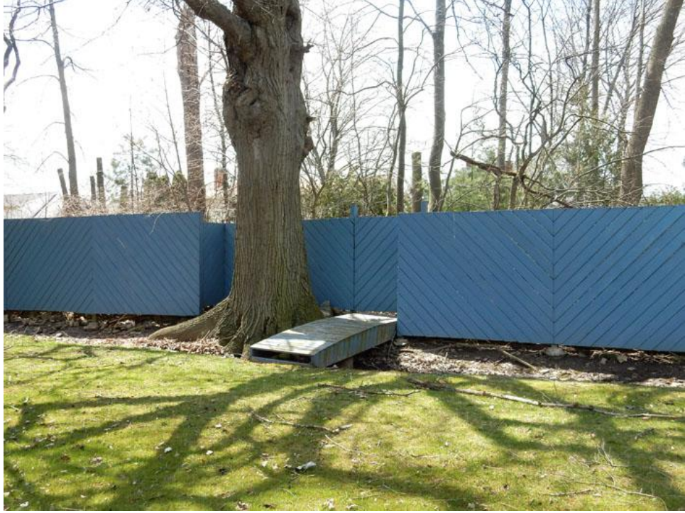
Figure93: 588 Charlotte Street, Wooden Replacement Wall
