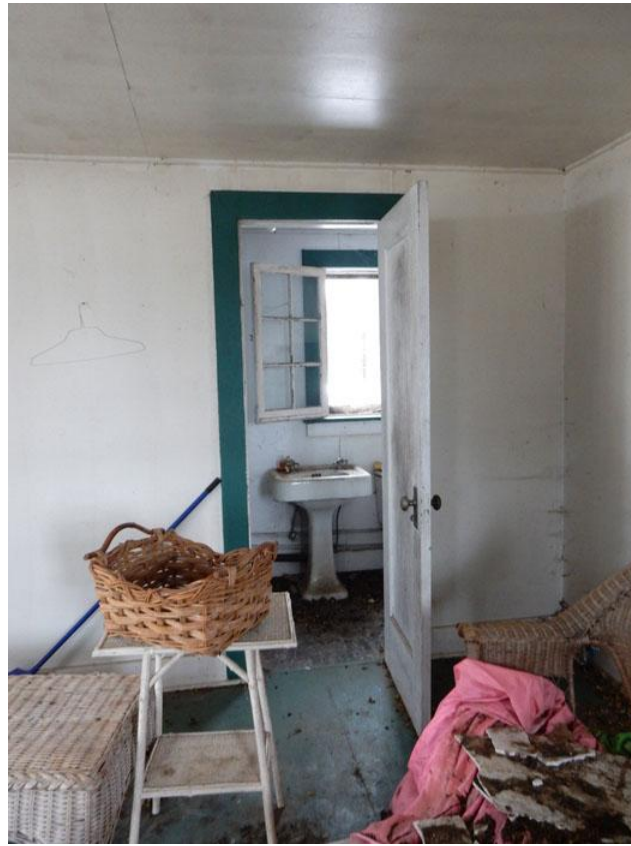
Figure55: 200 John Street, Pool House, View of Washroom
