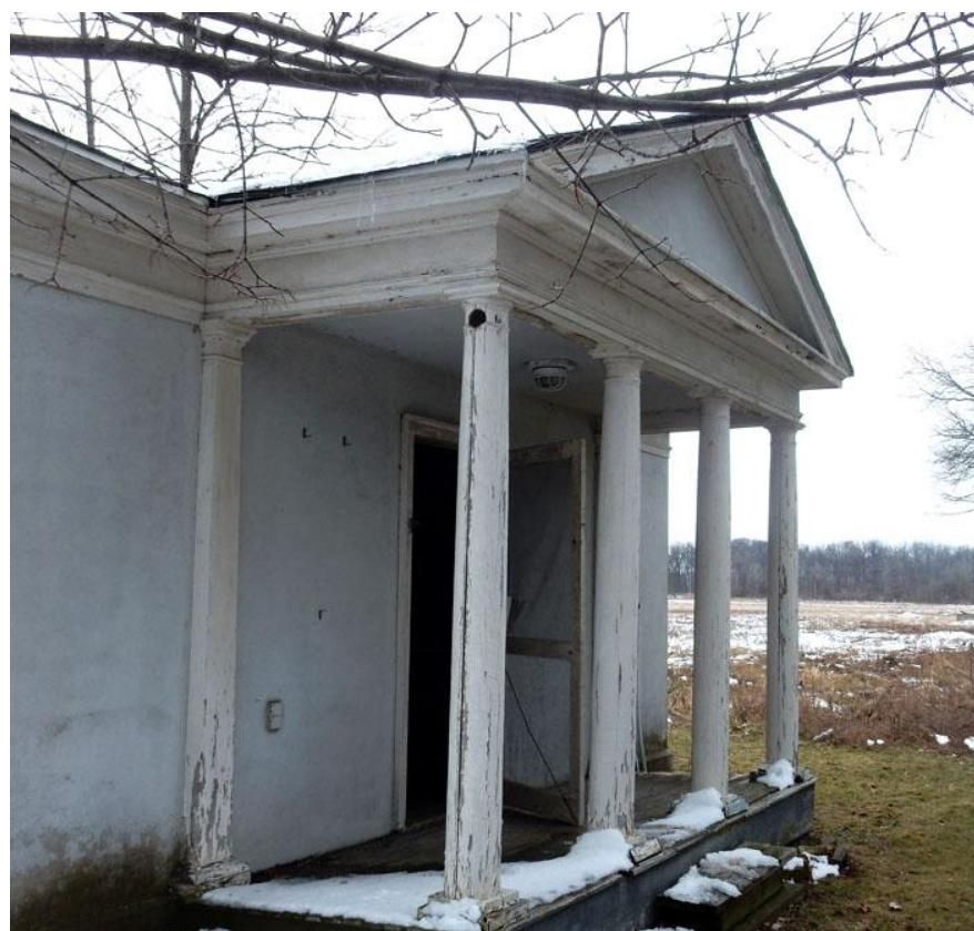
Figure 47: 200 John Street, Pool House, Portico
