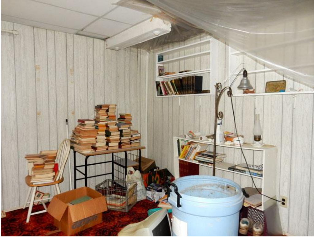
Figure34: 200 John Street, Garage Apartment, Bedroom Beaver Board Walls
