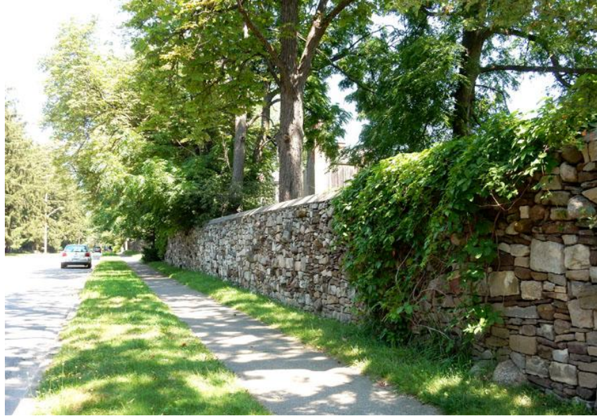
Figure 30: Stone and Concrete Wall along Charlotte Street Looking North
