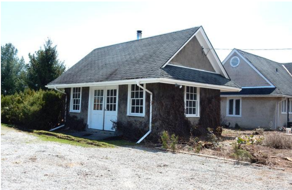
Figure84: 588 Charlotte Street, Outbuilding Two
