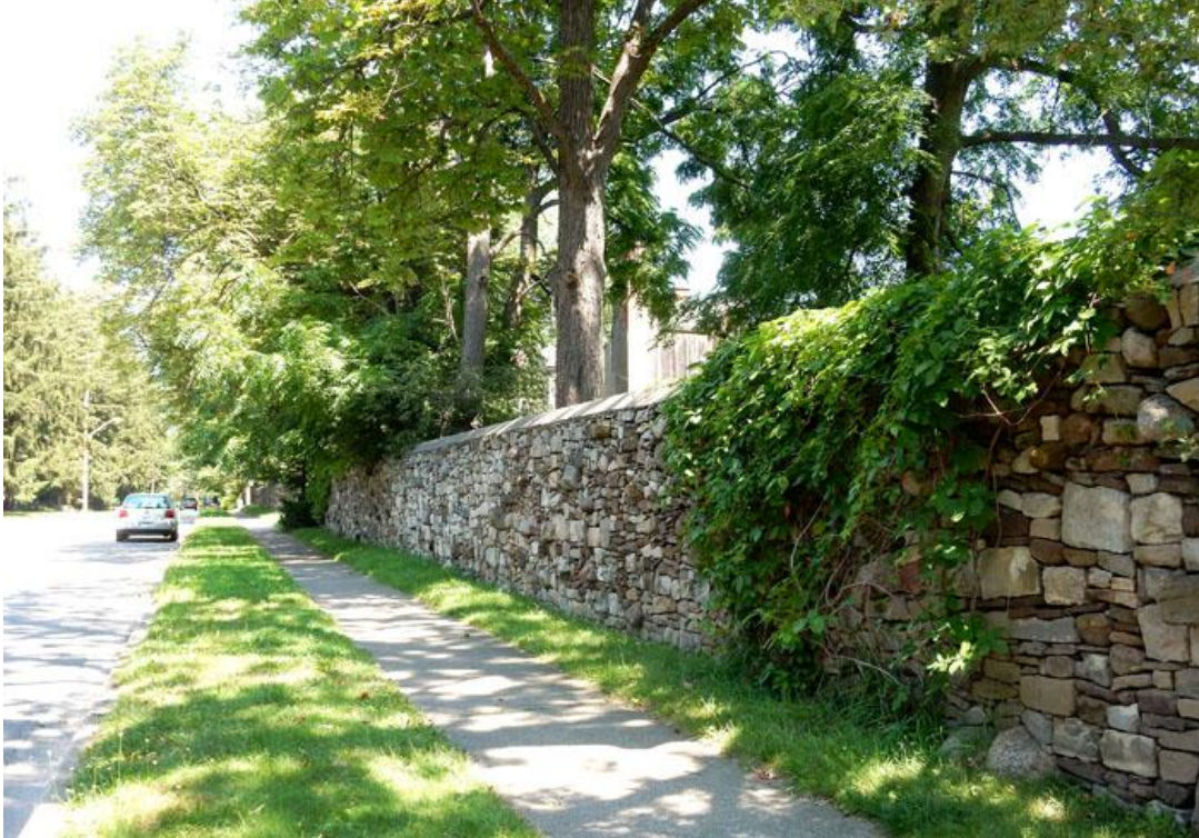
Figure 14: Charlotte Street Wall Looking North
