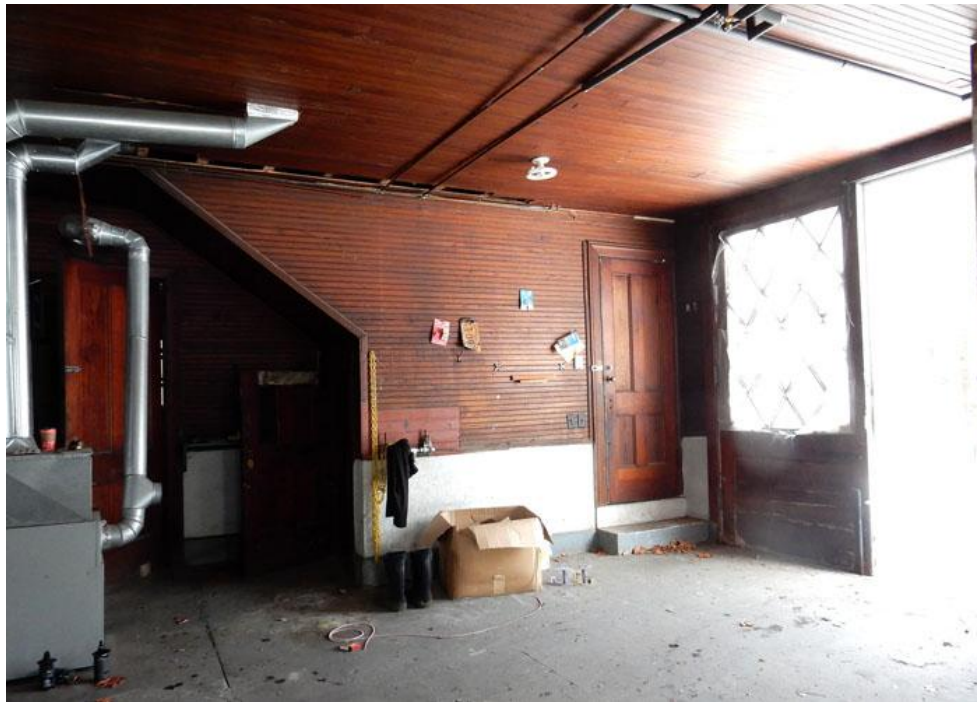
Figure 23:200 John Street, Garage, Ground Floor Looking West
