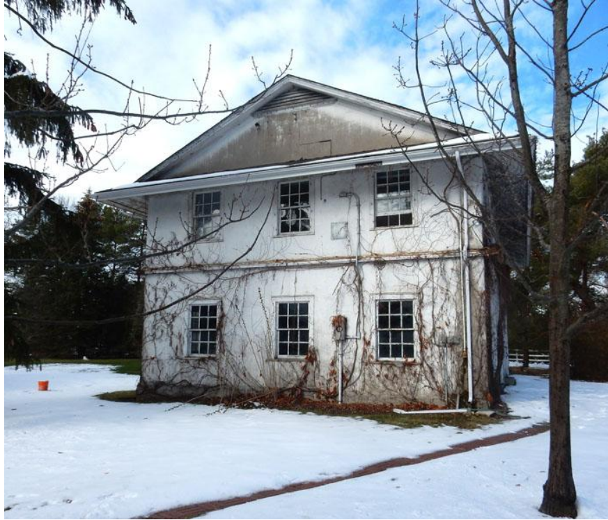
Figure20: 200 John Street, Garage, East Elevation
