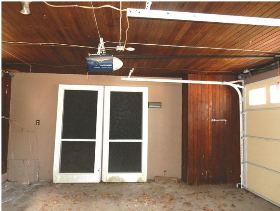
Figure 81: 588 Charlotte Street, Stables/House, Garage
