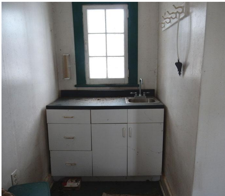
Figure 57: 200 John Street, Pool House, Kitchen Unit
