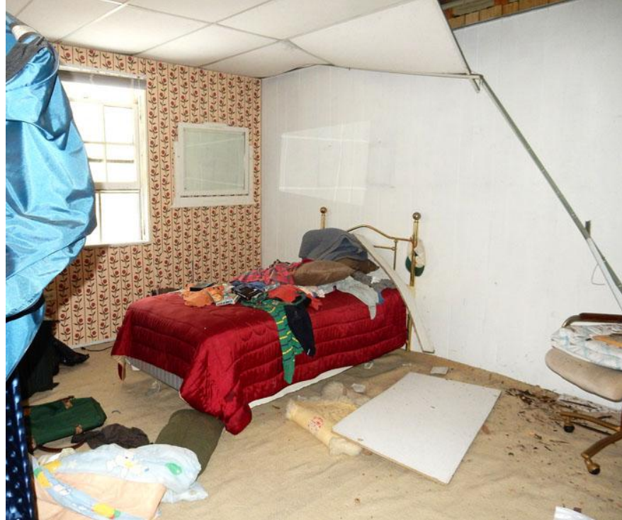
Figure32: 200 John Street, Garage Apartment, Bedroom
