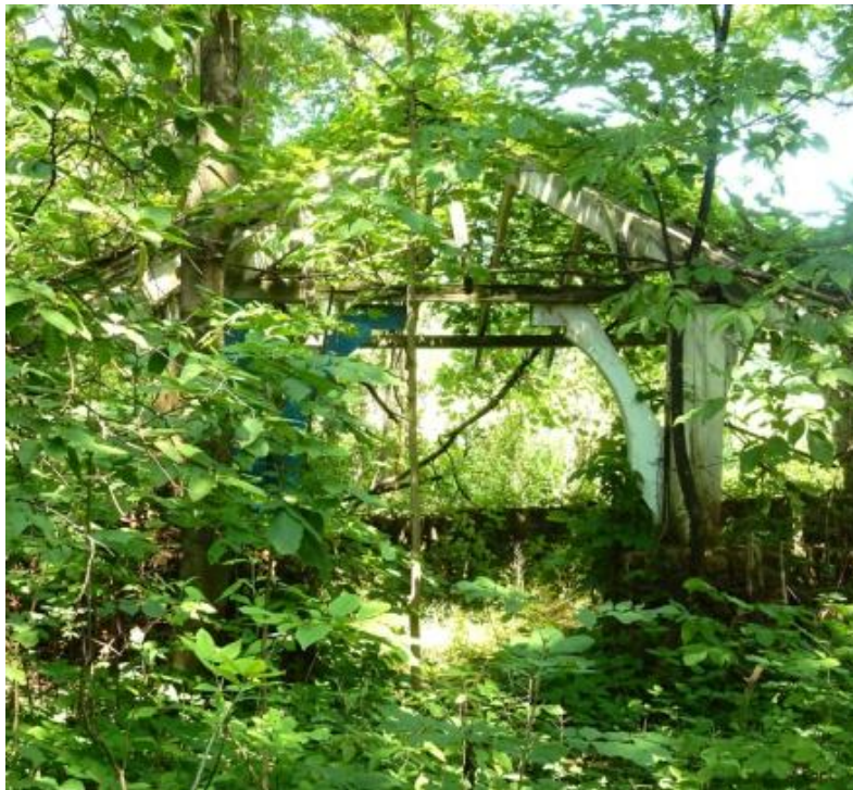
Figure24: Pergola at Rear of 200 John Street
