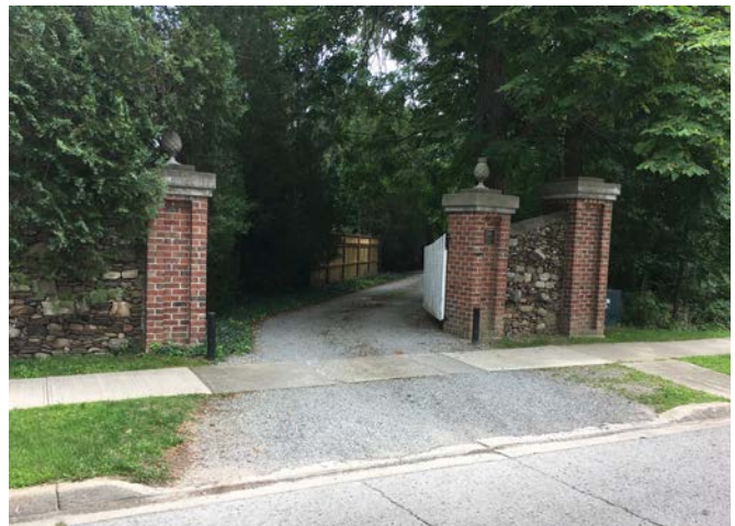
Image 4. Historical entrance to subject site from Charlotte Street
